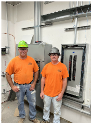
IBEW members Craig Matin and Adam Gillman working on Collins-Hammond project at Tim Hortons in Morristown.
